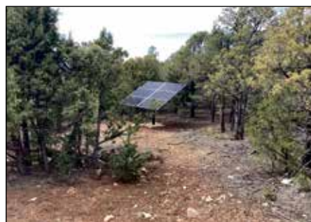
Pole-mounted PV panels in back yard.
