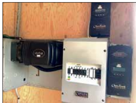
Inverter and charge-controller electronic components.
