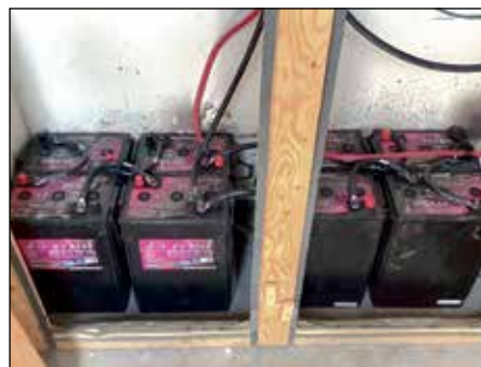
Battery bank of 16 sealed lead-acid heavy duty batteries. My next batch will be lithium ion batteries.
