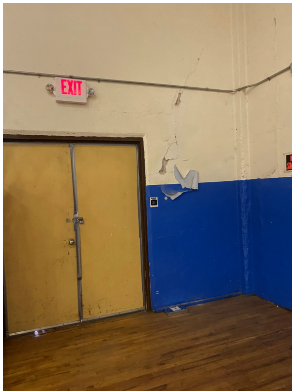
Photo 42 – Gym interior walls and ceiling at corner with visible water stains and cracks at SW corner.
