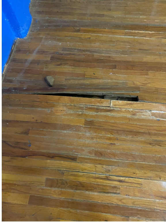
Photo 45 – Gym wood floor plank buckle and separation.
