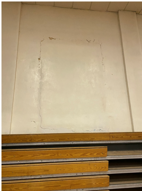
Photo 38 – Gym interior wall crack around previous window opening.
