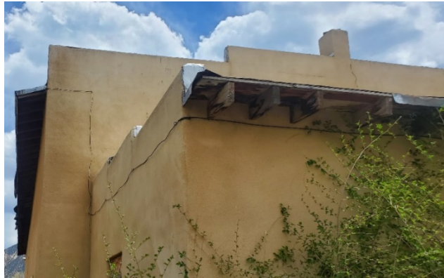
Exposed Framing and Roof Decking
