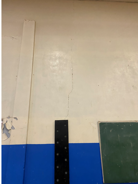
Photo 33 – Gym interior, cracks on interior masonry wall
