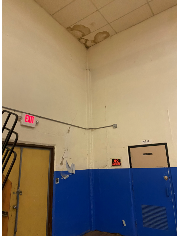
Photo 41 – Gym interior walls and ceiling at corner with visible water stains and cracks.
