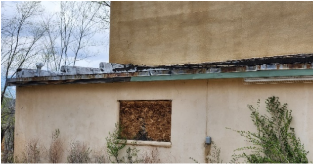
Fascia and Drip Edge Flashing, Parapet Patching
