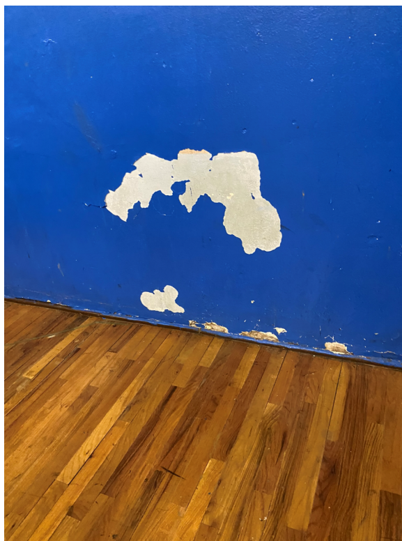
Photo 44 – Gym interior wall at floor with visible moisture damage.
