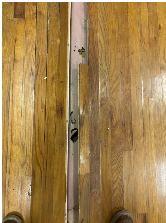
Photo 52 – Gym floor buckle and separation close-up view.
