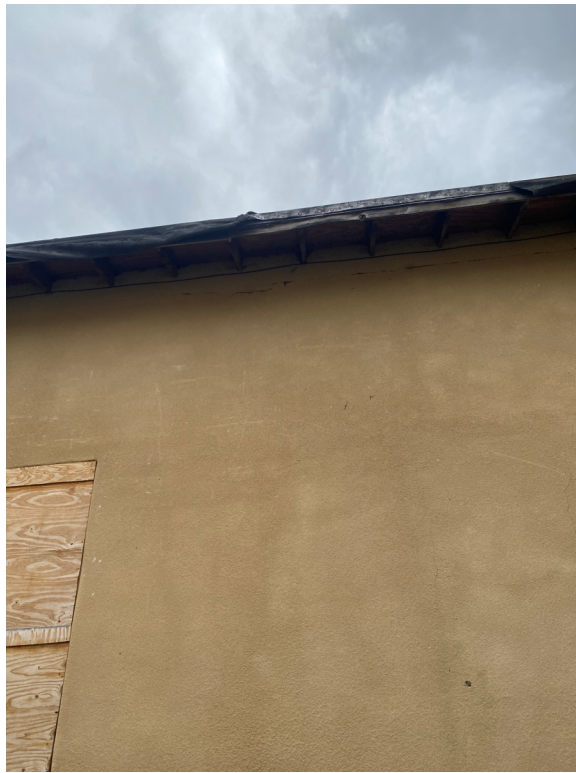
Photo 9 – Exterior building elevation with exposed soffit.
