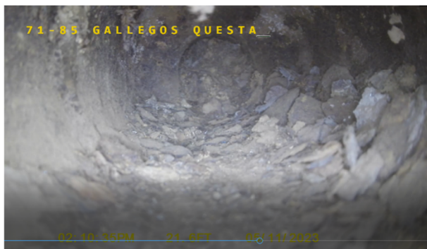
Blocked Sanitary Sewer
