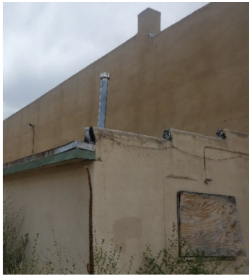
Parapet and Fascia Conditions
