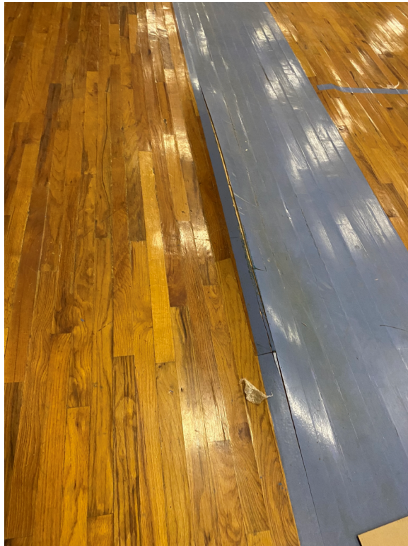
Photo 40 – Gym wood floor planks buckled, warped and uneven.
