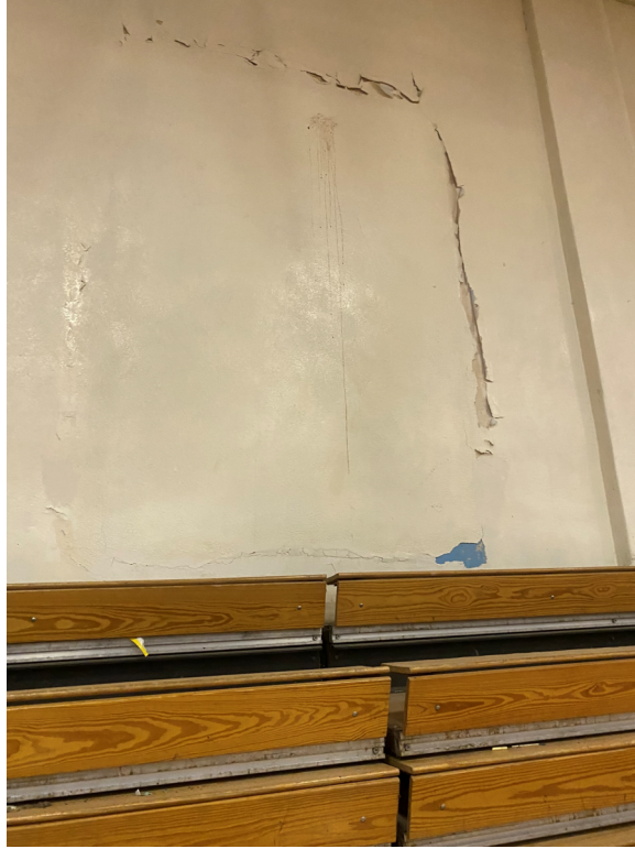
Photo 39 – Gym interior wall crack around previous window opening.
