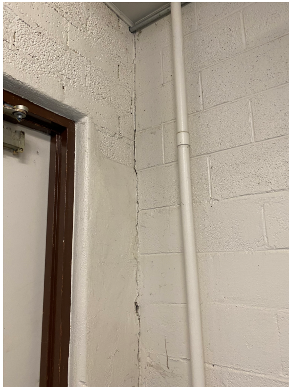
Photo 68 – Gym locker room masonry and brick wall at corner with crack.
