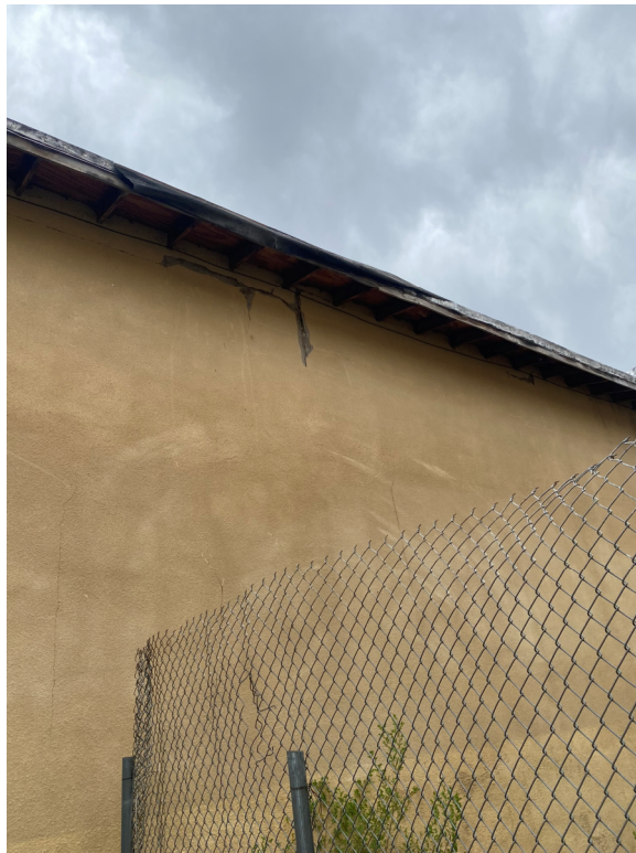
Photo 8 – North- West corner exterior building elevation with exposed soffit and visible cracking
