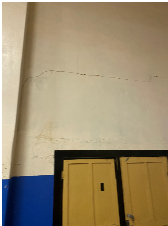
Photo 36 – Gym interior masonry wall cracks above doorway.
