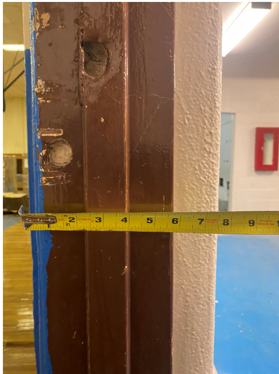
Photo 58 – Gym to locker room, 8-inch masonry wall.
