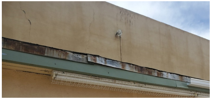
Fascia and Drip Edge Flashing, Parapet Patching
