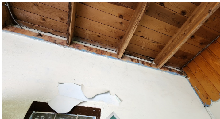
Entry Water Damage
