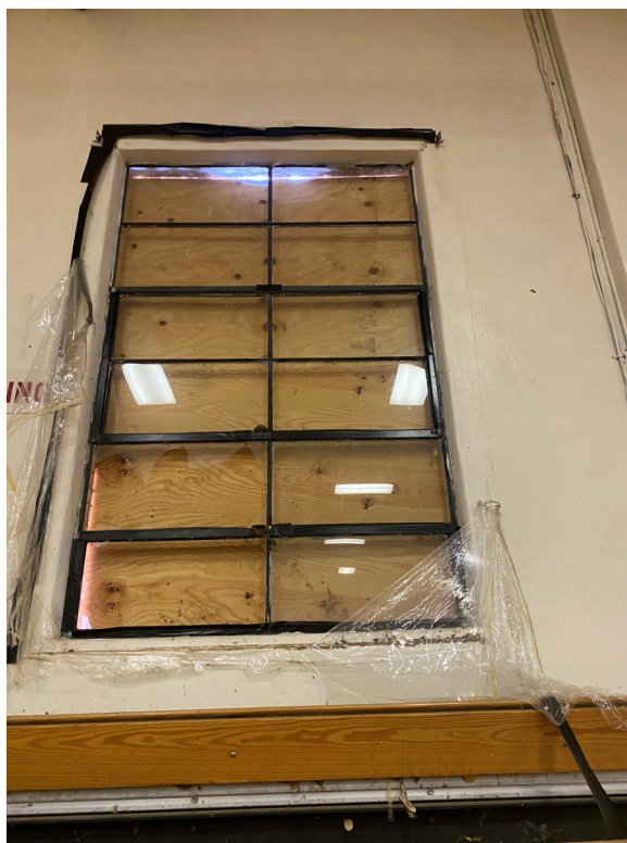
Photo 50 – Gym interior north wall with infilled window.
