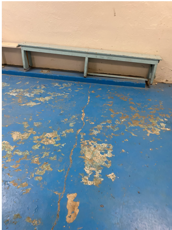
Photo 65 – Gym locker room concrete slab crack.
