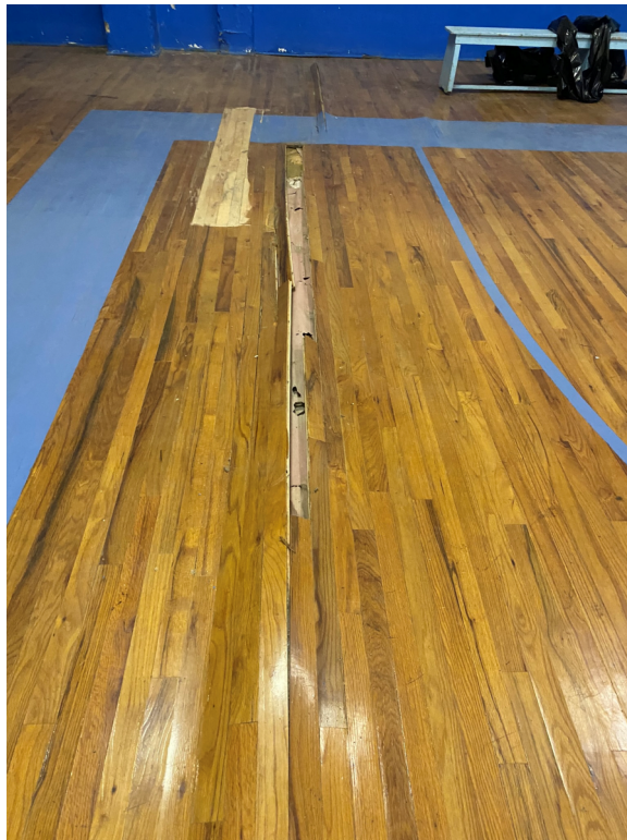
Photo 51 – Gym floor separation and buckling.
