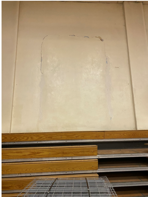
Photo 48 – Gym interior north wall with infilled opening.
