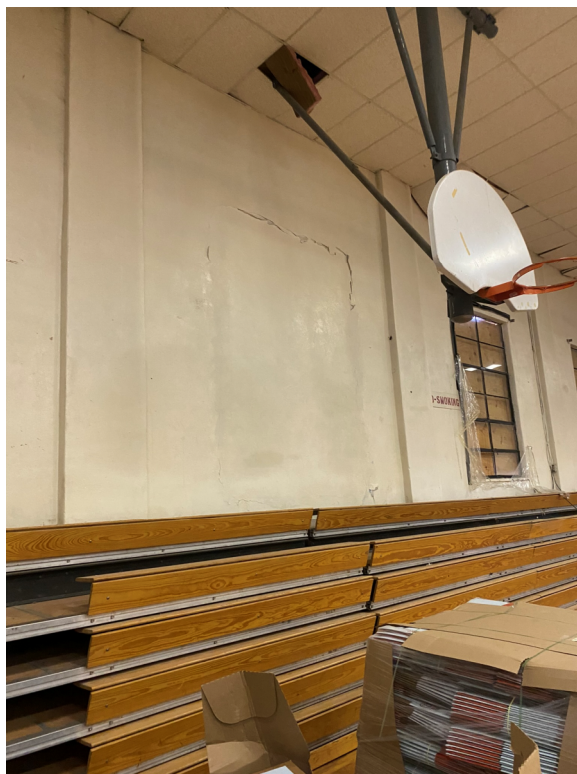
Photo 49 – Gym interior north wall at with infilled opening.
