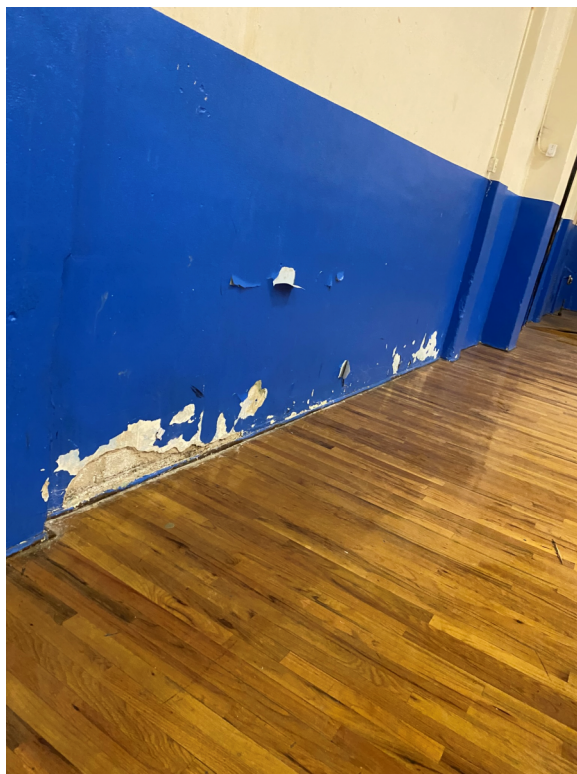
Photo 43 – Gym interior wall at floor with visible moisture damage.
