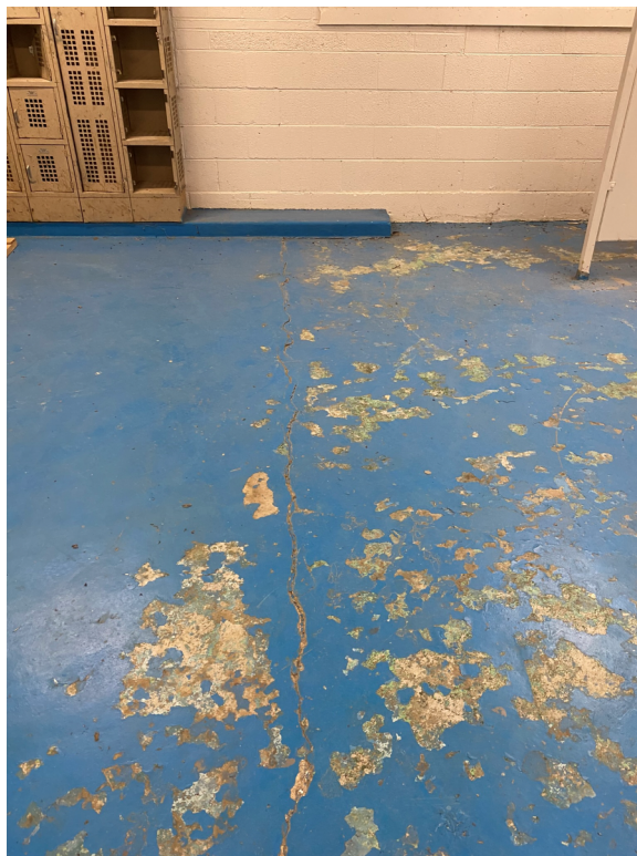
Photo 66 – Gym locker room concrete slab crack.
