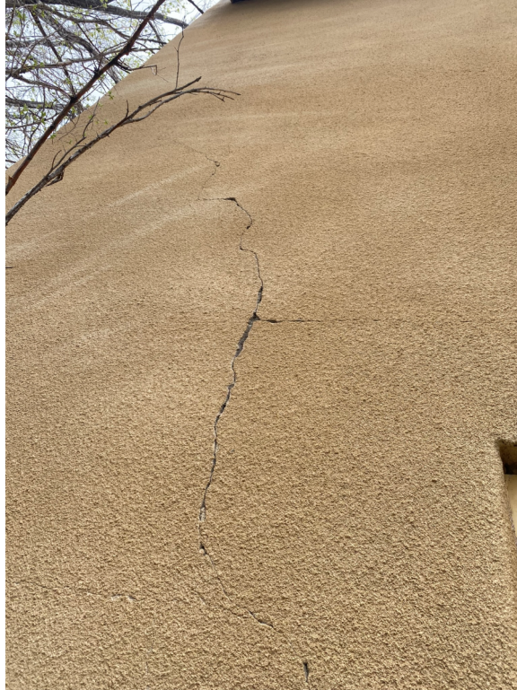
Photo 15 – Exterior wall stucco crack.
