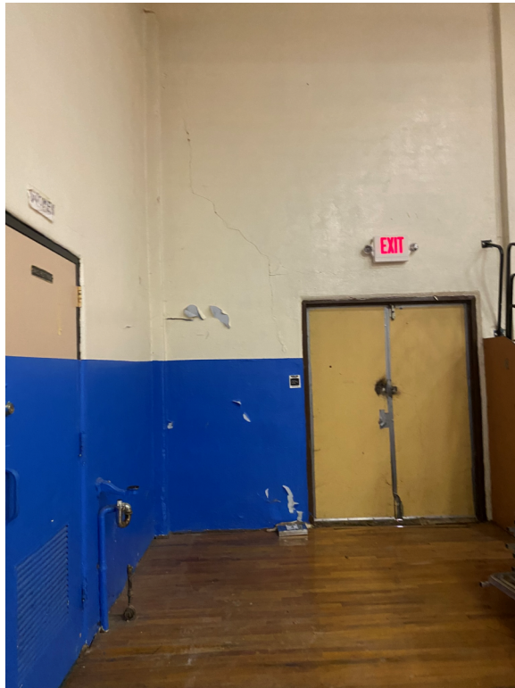
Photo 46 – Gym interior wall at NW door with cracks and visible moisture exposure.
